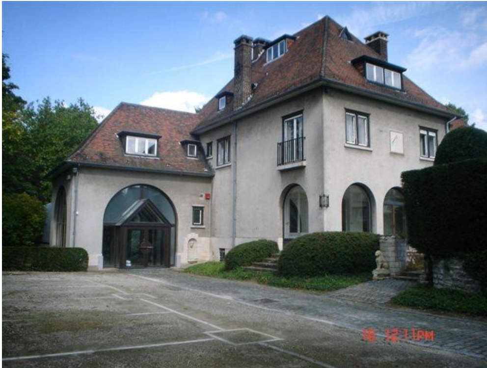
Main building 940 m 2
